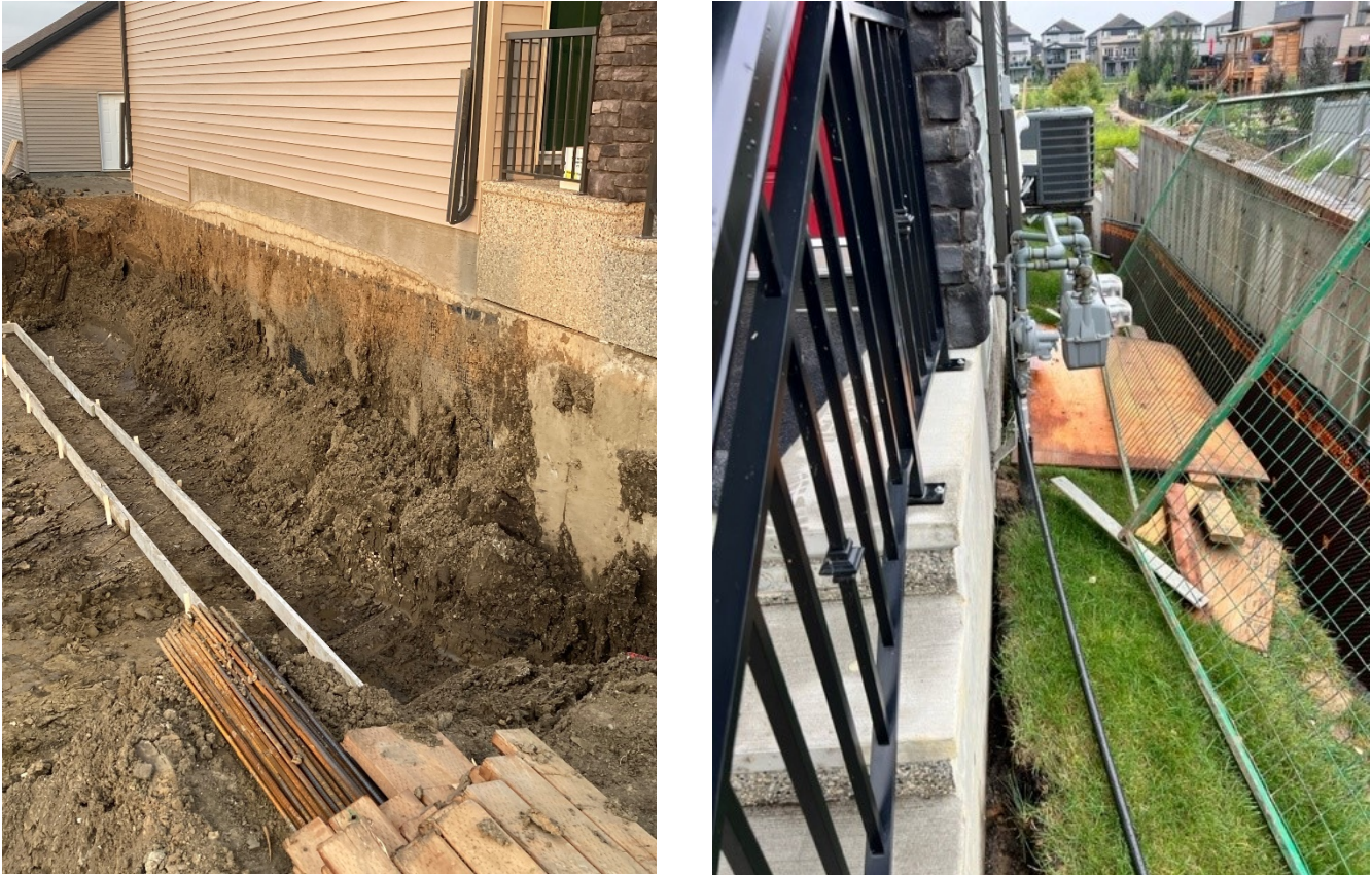
Figure 2: Foundation Excavation in Zero Side Yard developments
