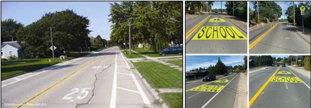
Figure 35. Sample Application of Pavement Marking Legends 3839
