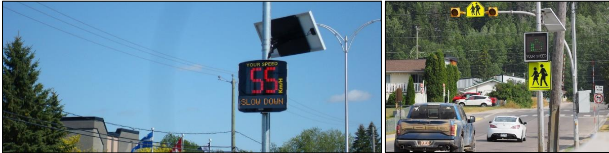
Figure 36. Sample Application of Speed Display Devices 4041
