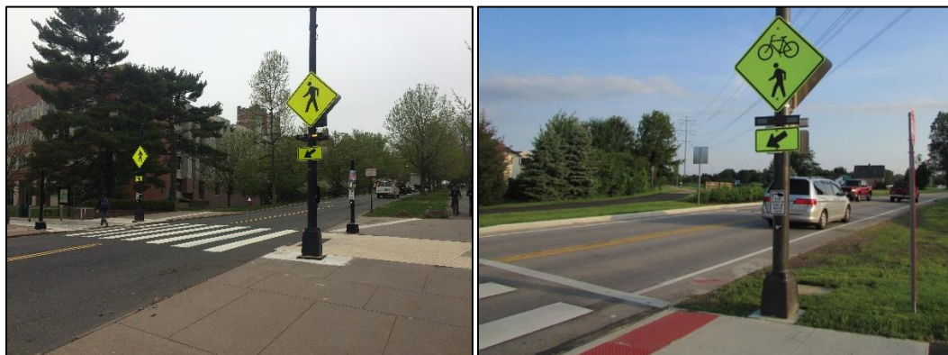
Figure 37. Sample Application of RRFB Equipped Crossovers
