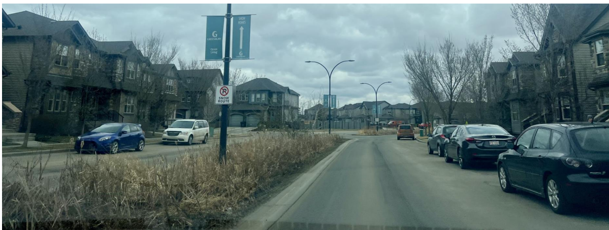
Figure 4.2 Greenbury Boulevard with street parking
