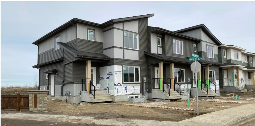
Rowhousing product under construction in Fenwyck
